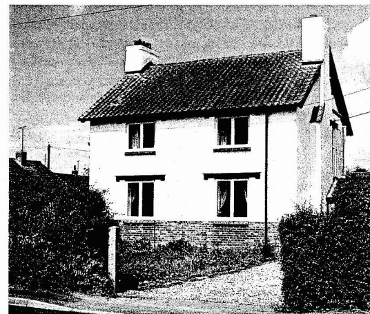
Figure 12. DSIR cottage in rammed chalk-cement at Amesbury, 1920.
