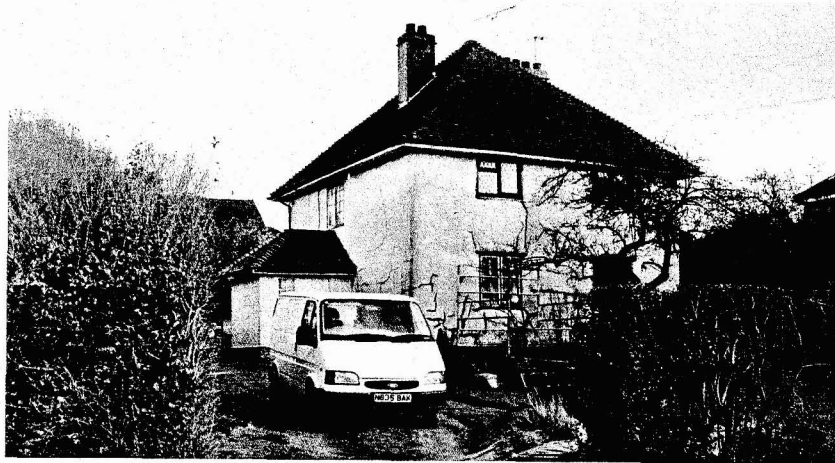
Figure 6. The first pisé cottage at Amesbury, built by the Board of Agriculture 1919-20.
